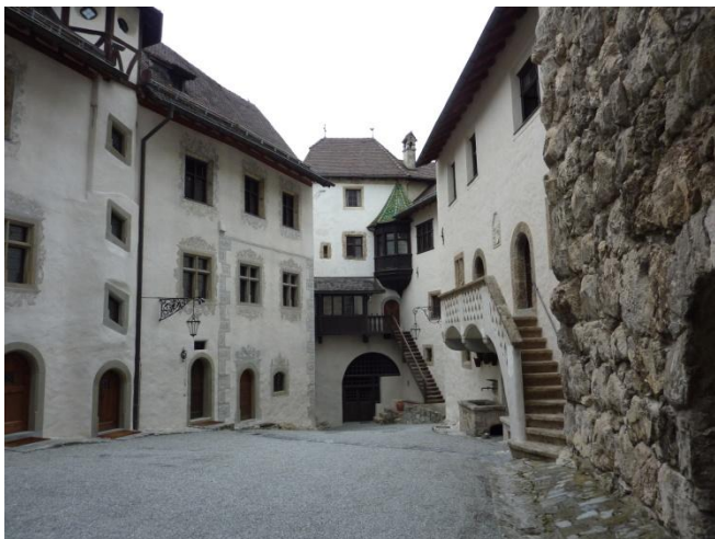
The third castle courtyard after its complete renovation, which took place between 2008 and 2011
