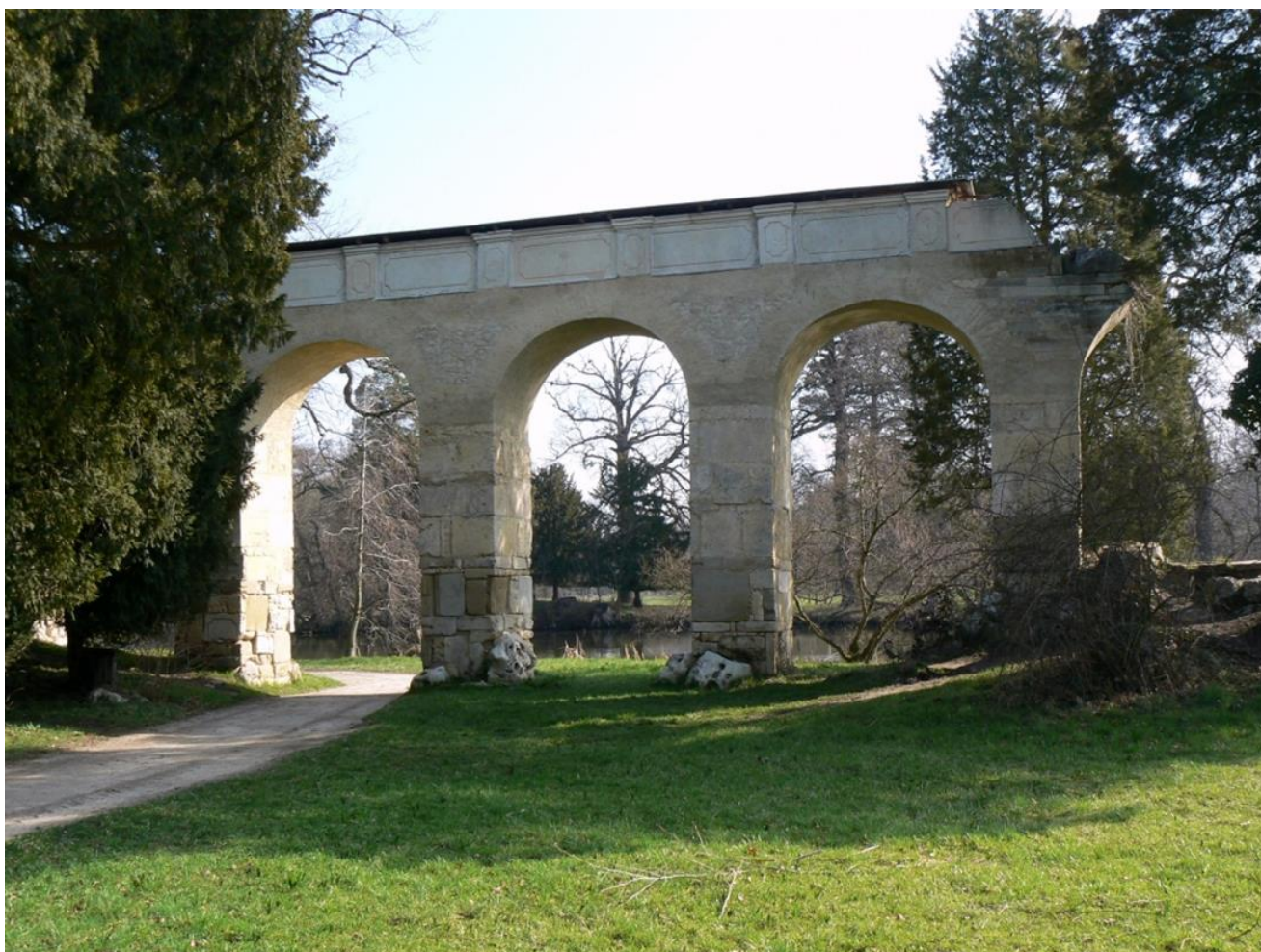
View of the repaired Roman aqueduct in the Lednice Castle Park
